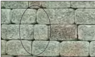
Avoid "stack bond" conditions where more than two courses create weak areas in the wall.
