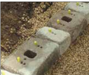
3. Insert Fiberglass Pins
