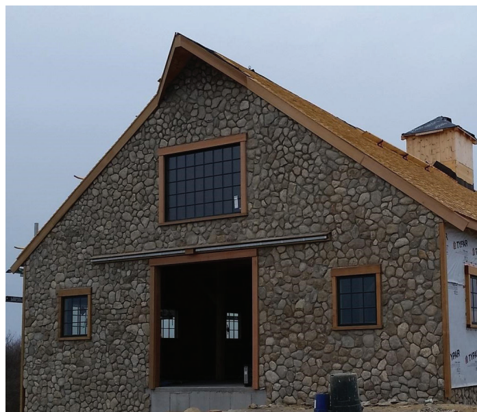
Top down installation with ARDEX X 77™ without mechanical supports
