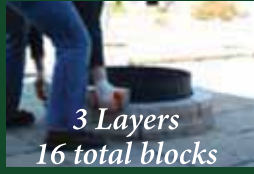
Set the ring and lay the blocks
