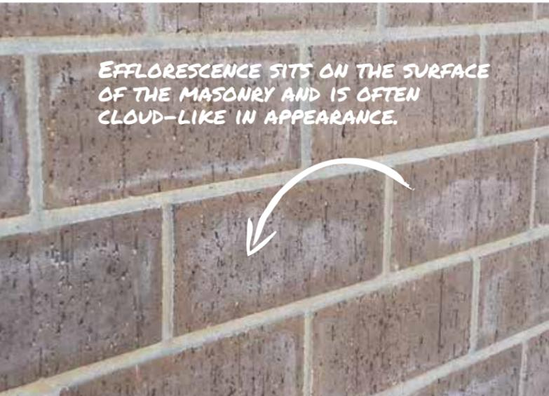
The result of soluble salts that already exist in the masonry coming into contact with water, acid or solvents, that then migrate to the surface of a masonry material through its pores.
