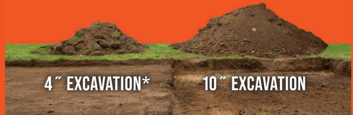
\*Final excavation depth will be determined by the paving unit thickness.
