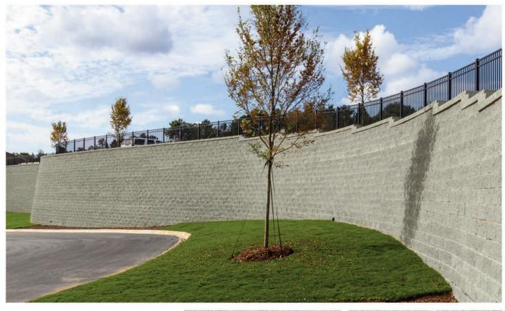
The 4 x  $2^{\circ}$  anchor bar on the underside of Premier 8 creates an automatic  $1^{\circ}$  (7°) setback with the highest shear resistance in the industry.
