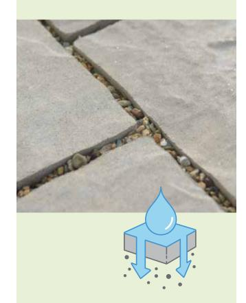
Permeable pavers look similar to traditional pavers but are designed with special spacer bars that create a wider joint.
