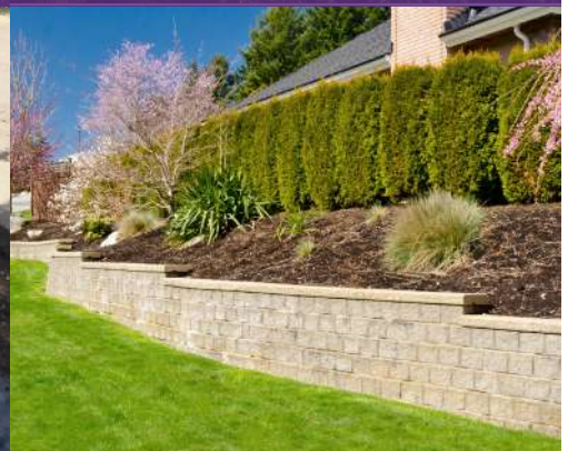
STABILIZATION FOR RET. WALL FOOTING
