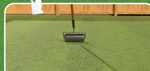
STEP SIX: Using a joint roller, firmly press turf evenly into the adhesive below
