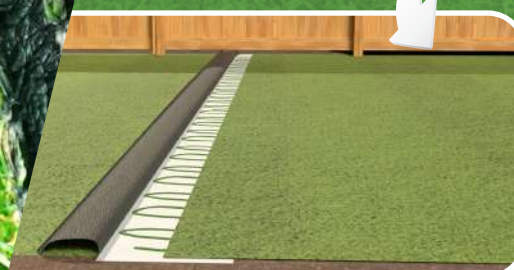
STEP FIVE: Align edges while pressing turf into adhesive
