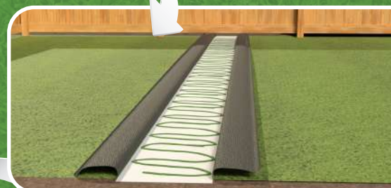
STEP FOUR: Apply Seams Right™ Turf Adhesive to the Seams Right™ Tape
