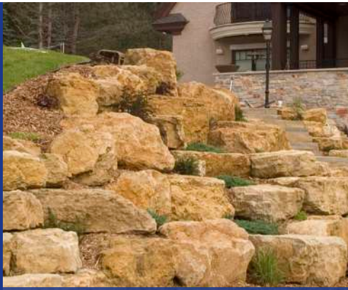
BOULDER RETAINING WALLS
